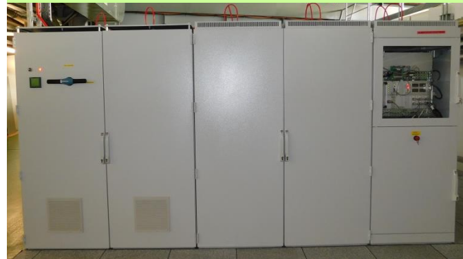
Spare SR sextupole & TL2 dipole power supply 50 kW
