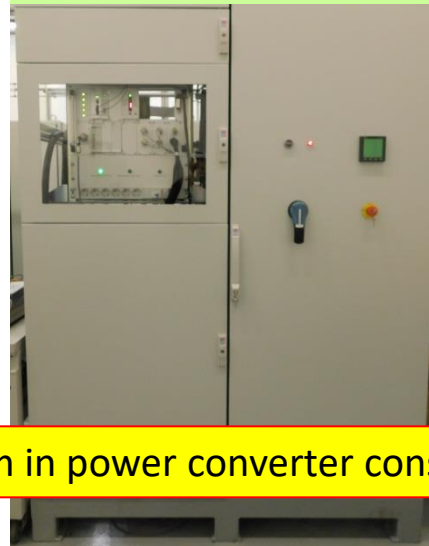
Spare SR sextupole & TL2 dipole power supply 50 kW
