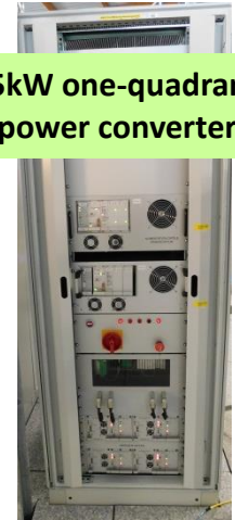
Spare SR sextupole & TL2 dipole power supply 50 kW
