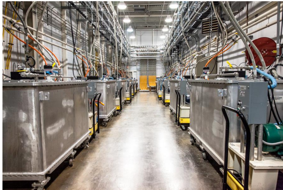
14 Extraction PFNs - Replacing Thyratrons with Solid-State Switches
