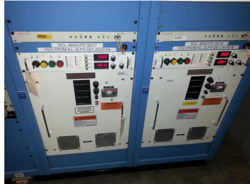
SCL Quads: Alpha Scientific 35V, 525A, PSI Controller
