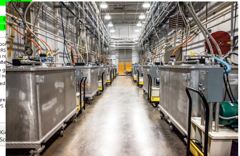
14 Extraction PFNs - Replacing Thyratrons with Solid-State Switches
