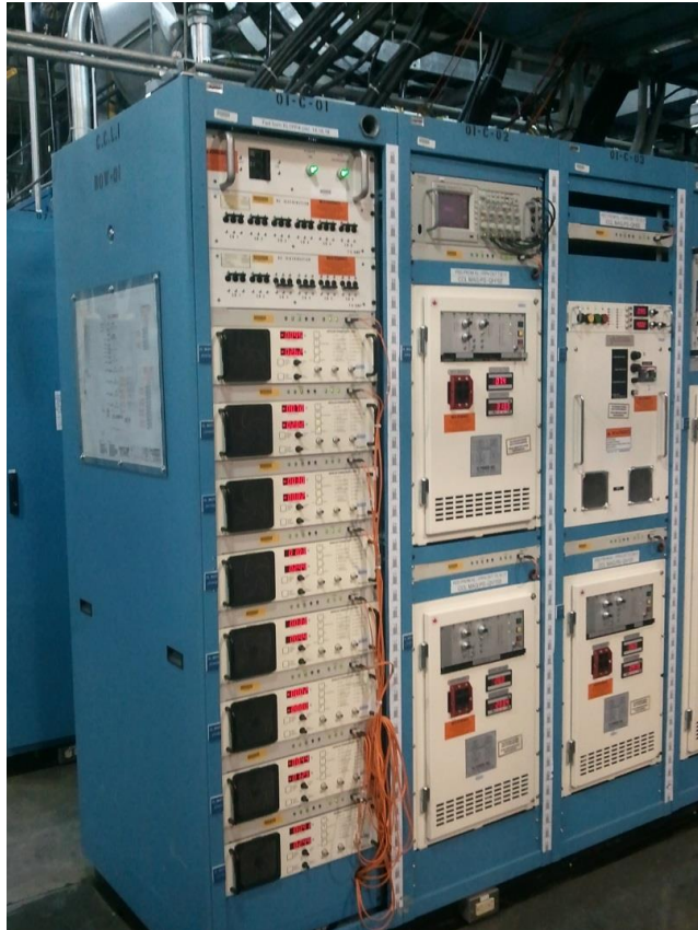
CCL Quads: IE Power Type II and III 20V-400A, 80V-375A PSI Controller
