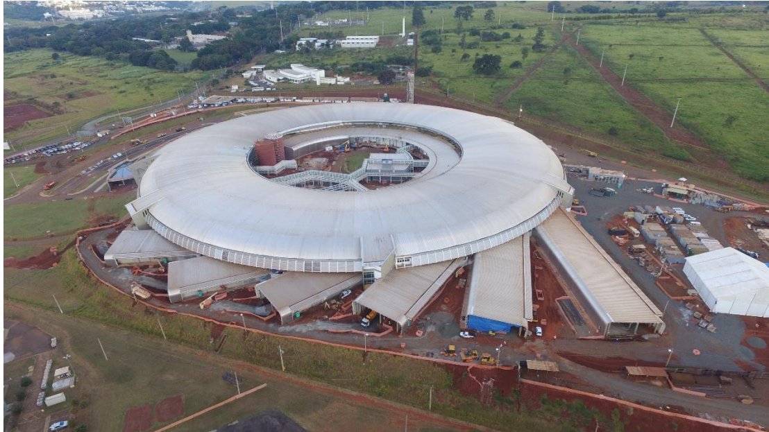
Sirius construction site, May 2018
