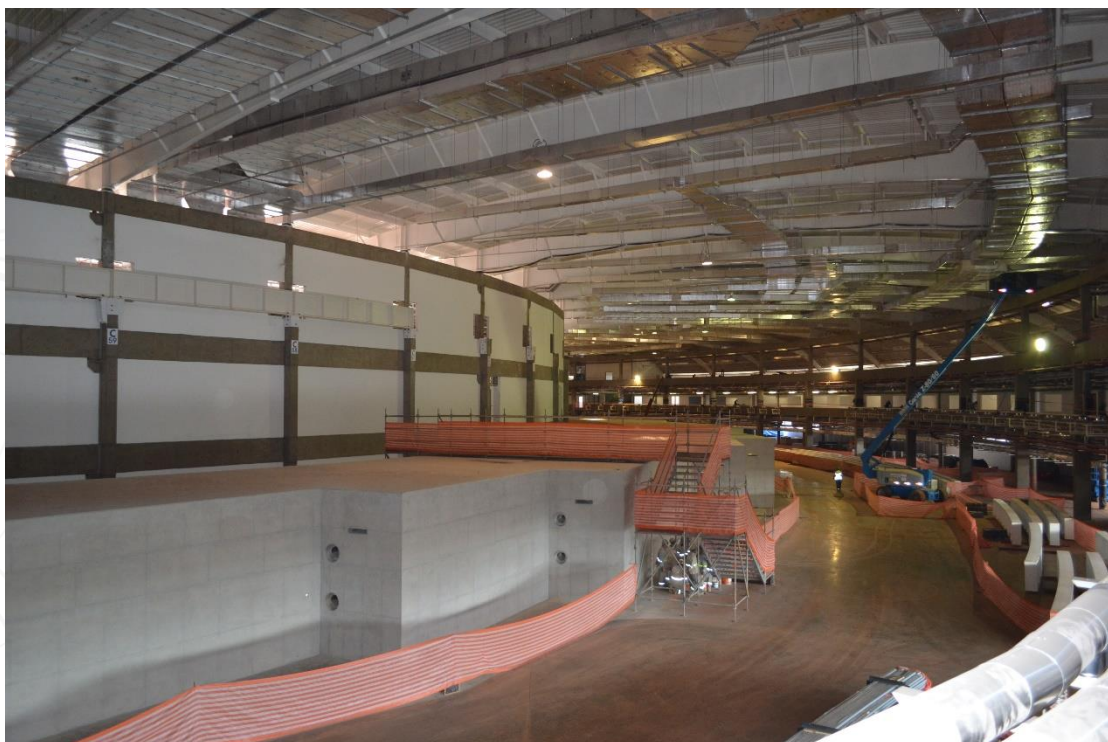
The experimental hall in construction, April 2018
