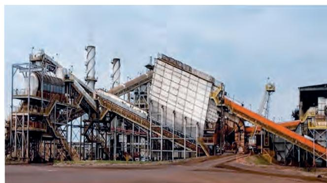
**Figure 51:** DCS with upward air blowing.
